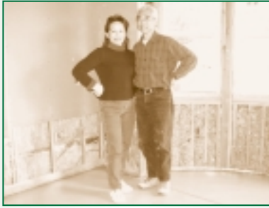
Bob & Lily Joe stand in front of a partially finished wall of their nearly completed Ecohouse. On the bottom left, you can see the exposed straw bale wall. On the bottom right, the wall insulation beneath the window is made from recycled denim.
